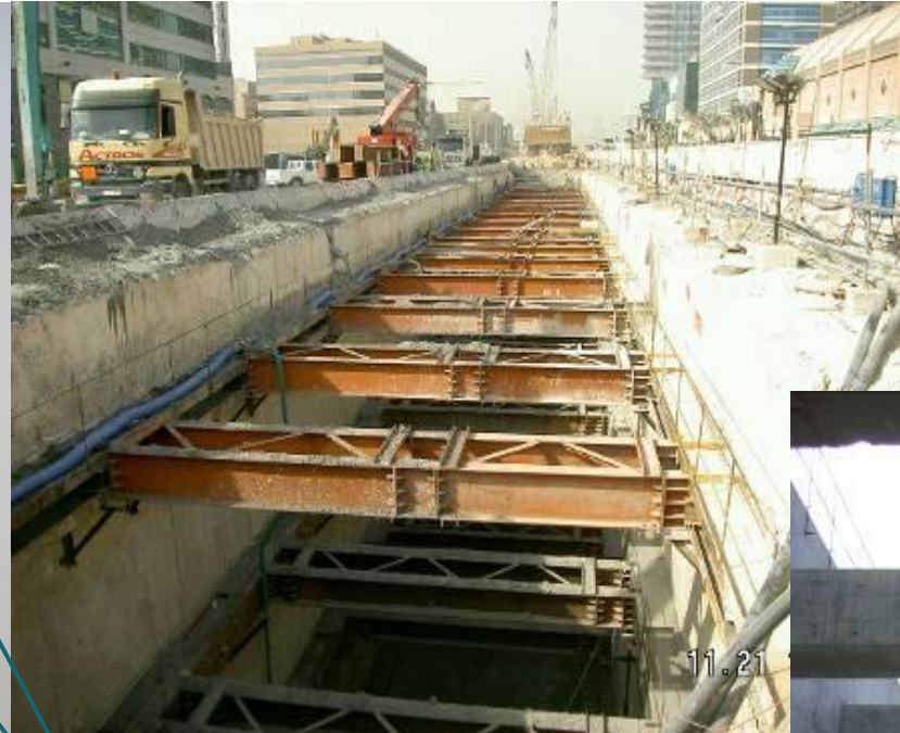
Multi-level strutting
