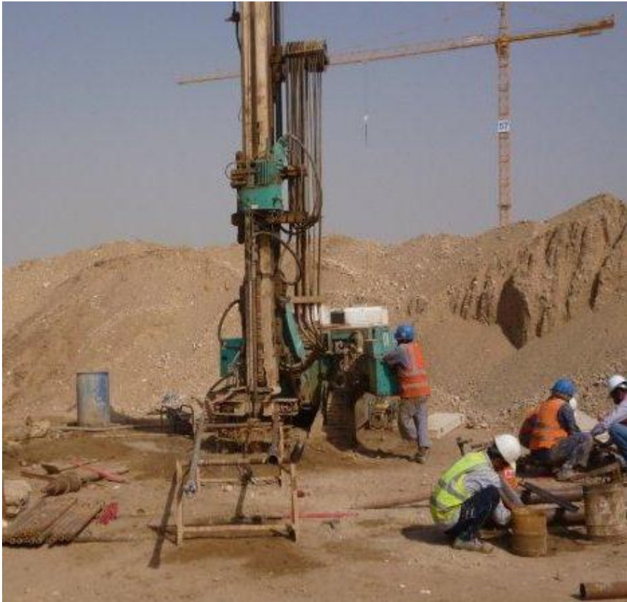
Rotary coring using double tube core barrel
