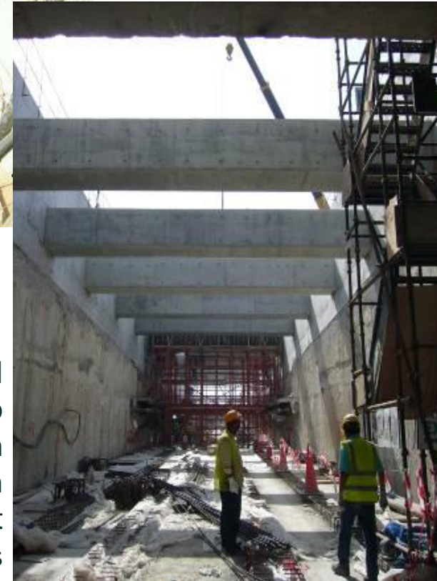
Tunnel portal to trough section with permanent RC struts
