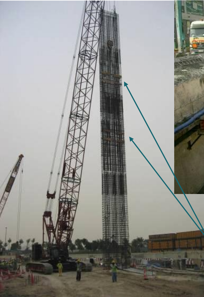
Diaphragm wall reinforcement cage being lowered into cut wall slot
